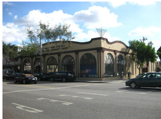
L'Chaim is one of 300 centers throughout California that will be affected. Credit Rhett Nadolny
